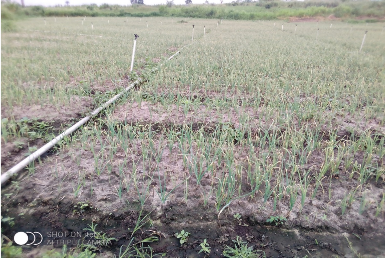
Construction of Irrigation Facility at Hwidiem (DACF)
