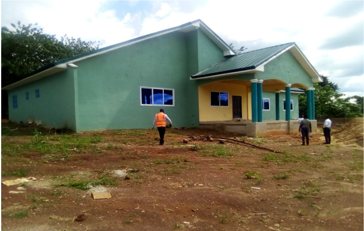
Construction of DCE's Bungalow at Hwidiem (DACF)
